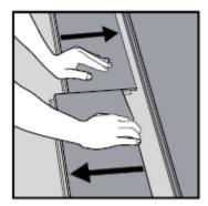
Separate the whole row by lifting it up delicately at an angle. To separate the planks, leave them flat on the ground and slide them apart.
